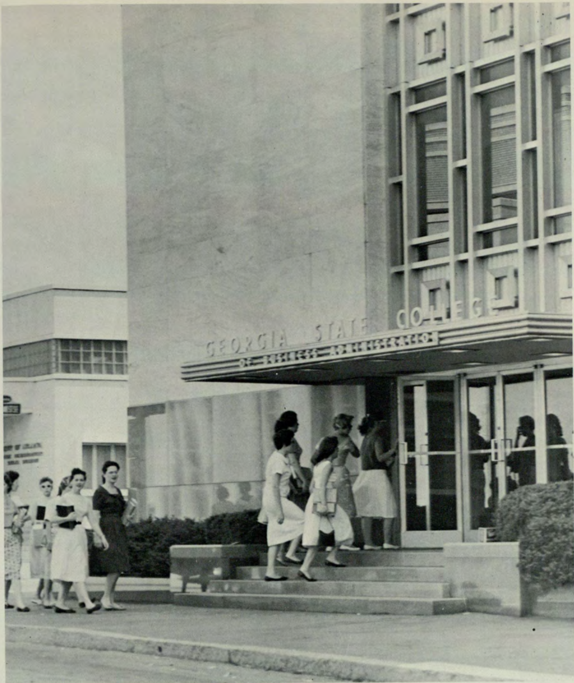
Main entrance on Gilmer Street
