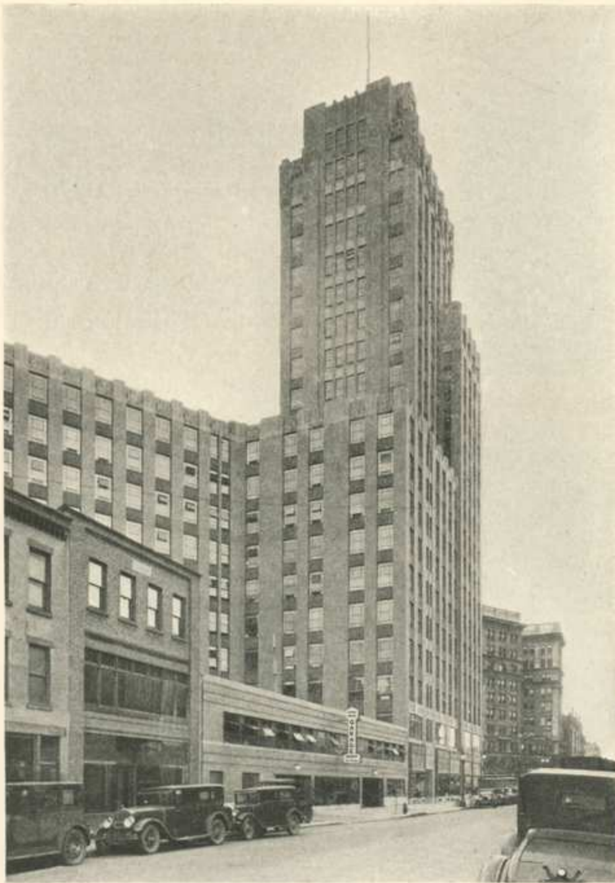
(At the left) State Tower Building, Syracuse, N. Y., again illustrates the combination office building and garage. The latter with two basement levels in addition to the above ground storage floors holds 140 cars.
