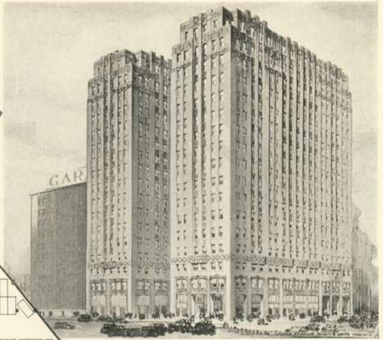
(Above) Medical Arts Building, which is part of the Cleveland Terminal Development, has a ten-story 1200 car garage as an annex to the office building proper. Note the adaptation of d'Humi Motorramps to the odd shaped garage portion of this building.
