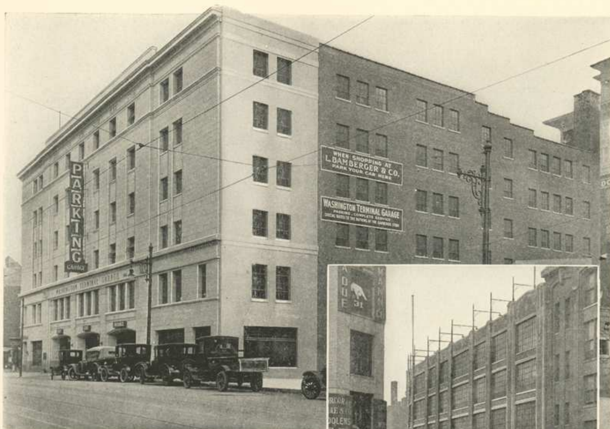
(Above) Washington Terminal Garage, Newark, N. J. serving the patrons of L. Bamberger & Co. MARSHALL N. SHOEMAKER, Arch't.
