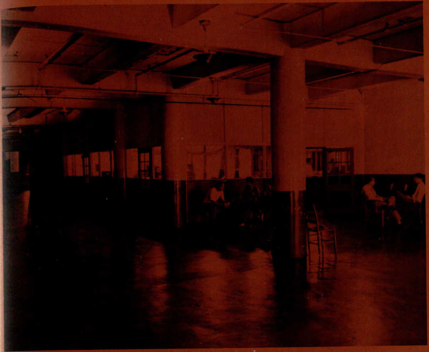
INSIDE THE BUILDING
