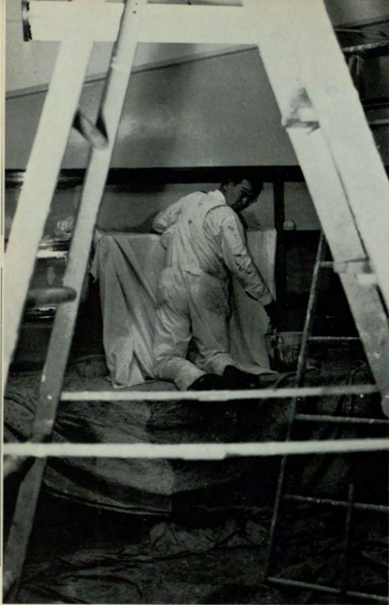
Rampway office gets a new face.
