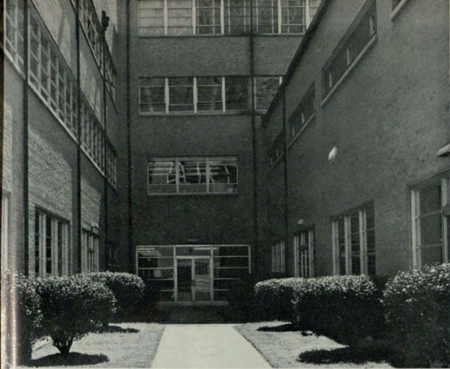
Sparks Hall from the patio.
