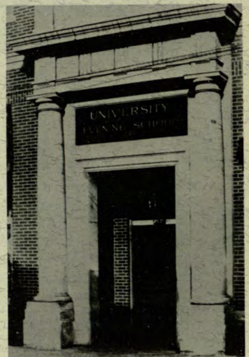
Detail of Entrance to 223 Walton Street Building.
