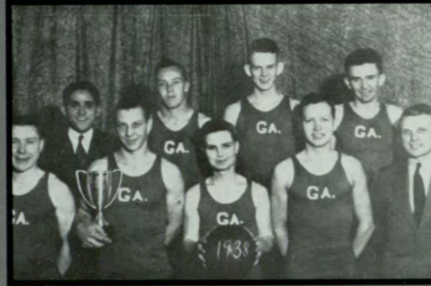
Below: Major Lathem's 1938 Basketball team. Bottom: The Urban Life Building under construction in 1973.
