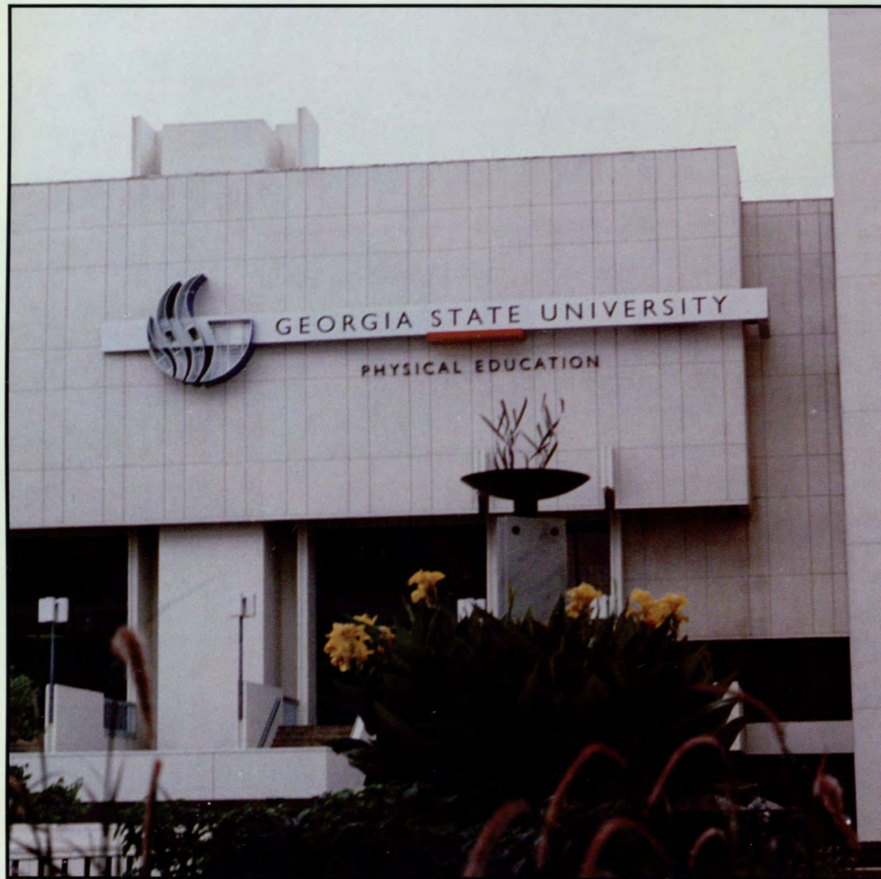
N ew signage around campus displayed Georgia State to viewers from around the world who were watching the Olympics on television. Signs were also installed on the One Park Place South building and on the Olympic Village. Photo by Jennifer Bebnke.
